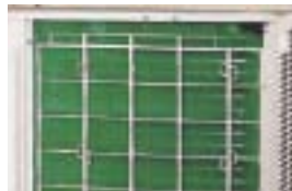
Green anti-corrosion coating pictured.
